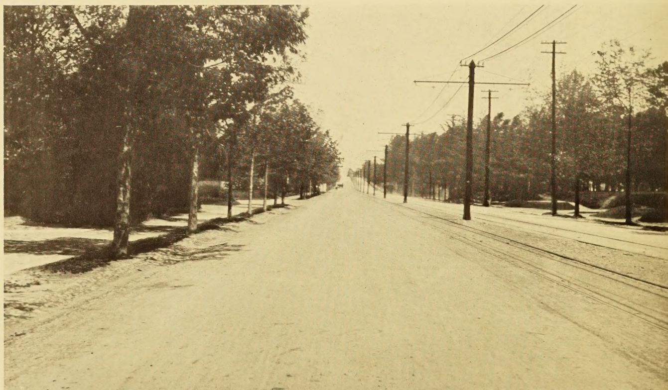
SURFACE CONDITION OF BITUMINOUS MACADAM SECTION IN MAY, 1912. THE PHOTOGRAPH ON THE FRONT COVER WAS TAKEN AT THE SAME LOCATION
